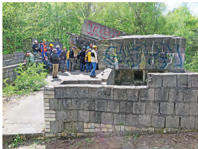
Block walls rise above the remnants of the Koralle briefing bunker and AA site. Photo Clive Penfold
